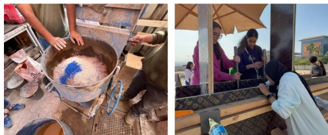
Fig. 6. Phase III 1:1 implementation. Part A Mixing the Earth, Part B Students ramming. (Source: Authors).
