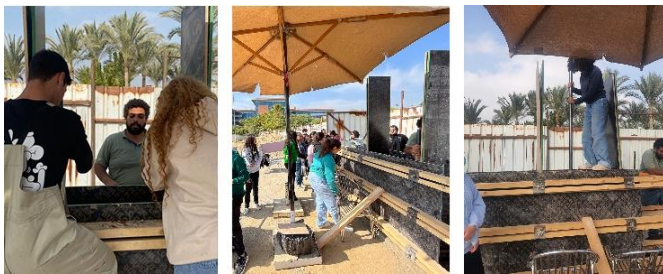
Fig. 15. Ramming process in 1:1 implementation (Source: Authors).
